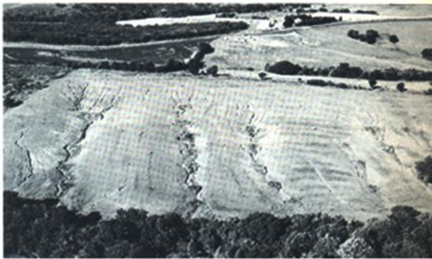
Fig 2.1 Erosion by sheet flow
