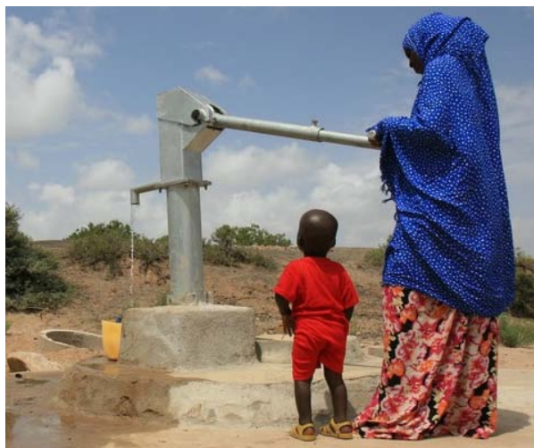
b) The lift pump in action
